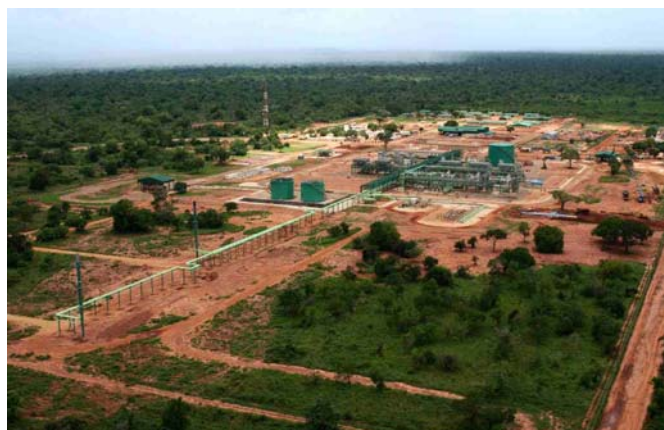
Central Processing Facility at Temane
