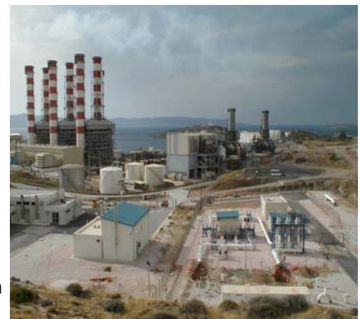
Lavrio Metering Station
