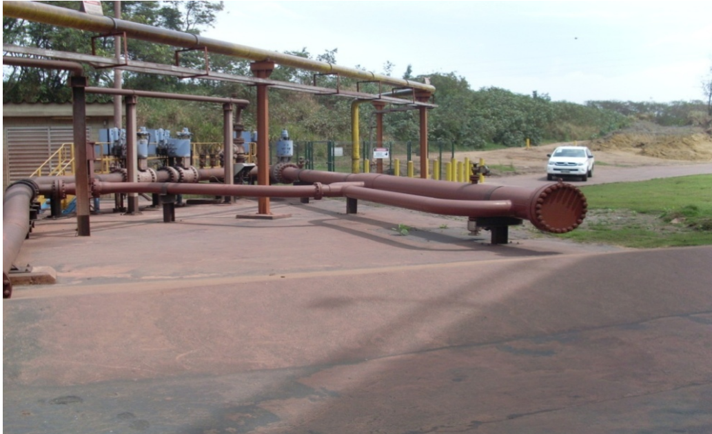
Figure 2. Pig Trap for a long inspection pig
