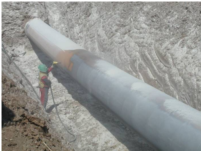
Figure 9 Blast cleaning in-situ on a large diameter pipeline (photograph courtesy Copon)
