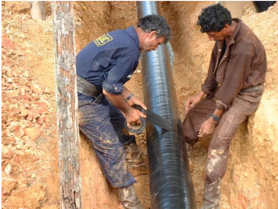
Figure 7 Field Applied Tape Coating
