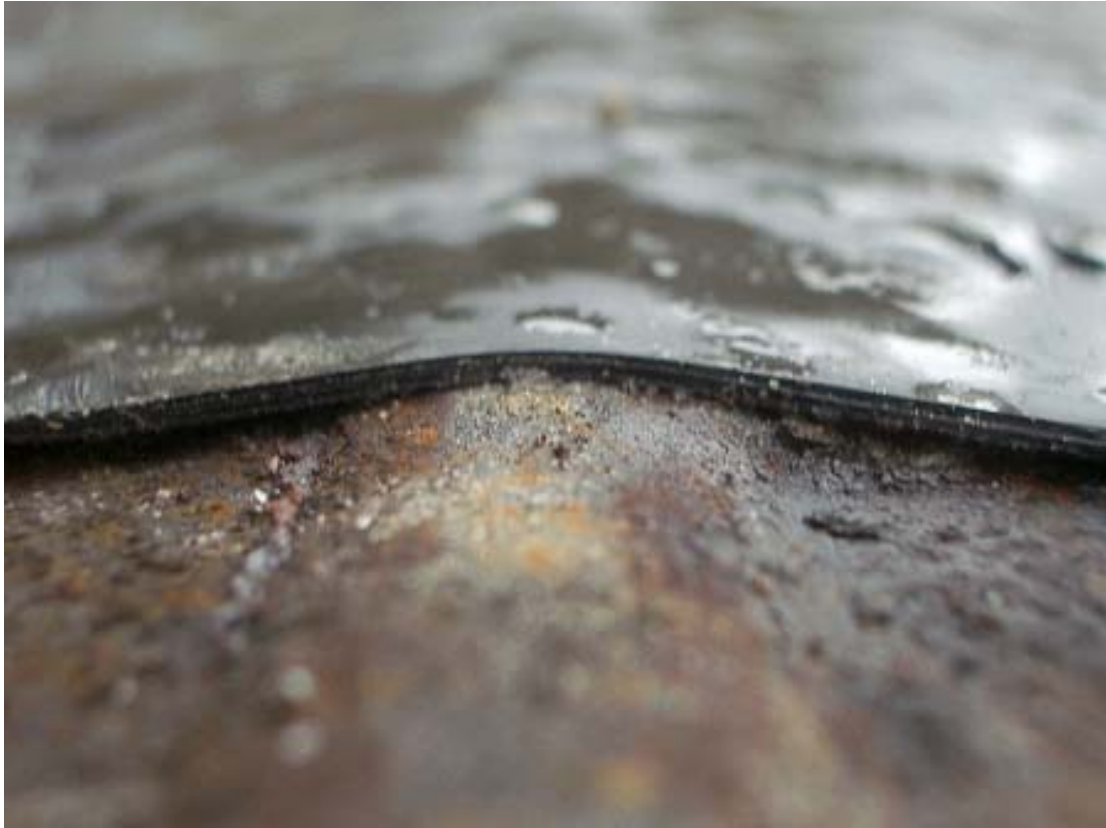
Figure 3 Tape Coating Tenting at Seam Weld
