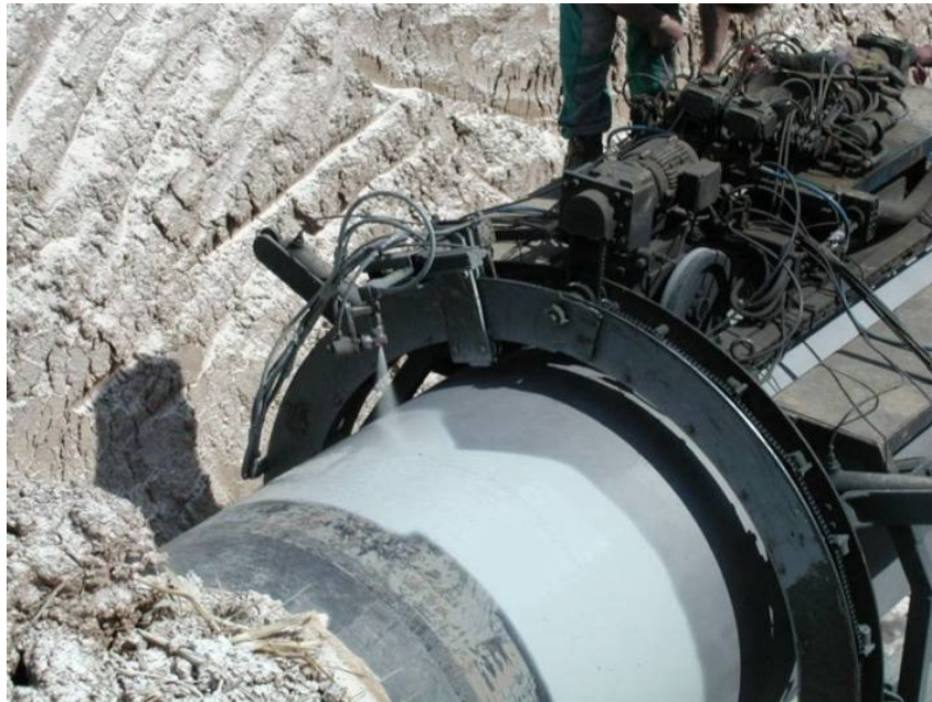
Figure 10 Automated Coating Application (photograph courtesy Copon)
