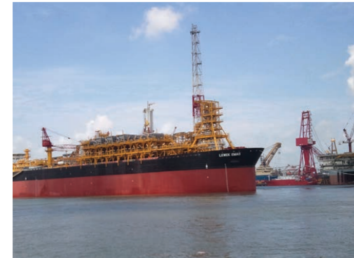
PHOTO: Lewek Emas FPSO Sector: Offshore FPSO/FPU Client: Premier Oil Location: Vietnam Services: Engineering and Project Management
