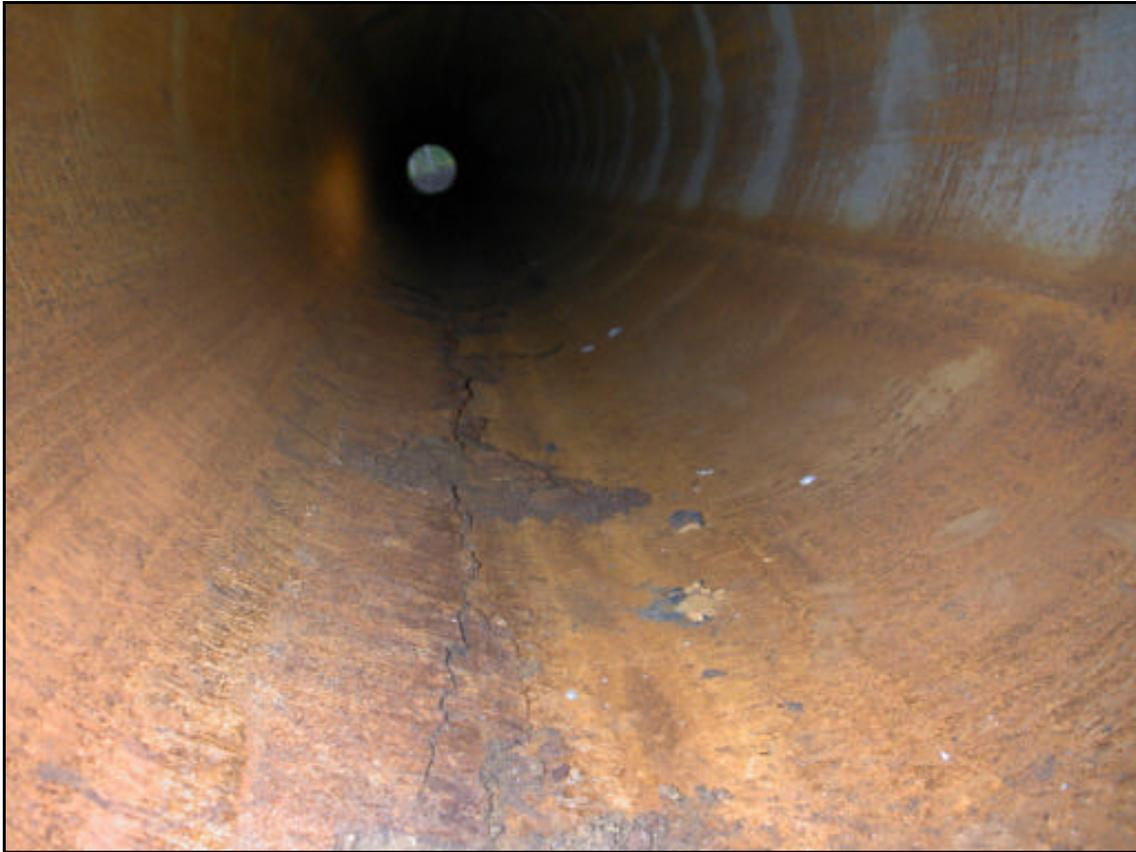
**Figure G1 – Debris Crust in the Bottom of the Pipe**
