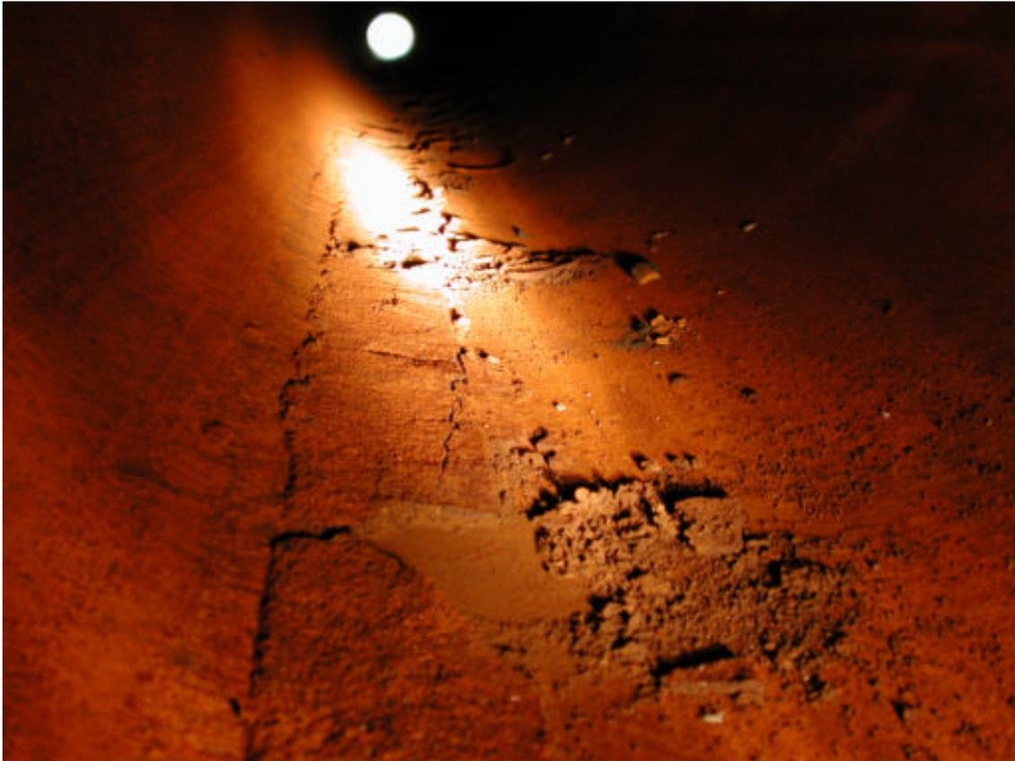
**Figure G2 – Debris Crust in the Bottom of the Pipe**
