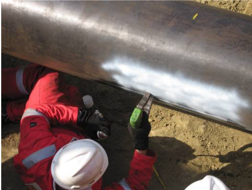
Figure 5 Typical Site Inspection (Magnetic Particle Inspection)
