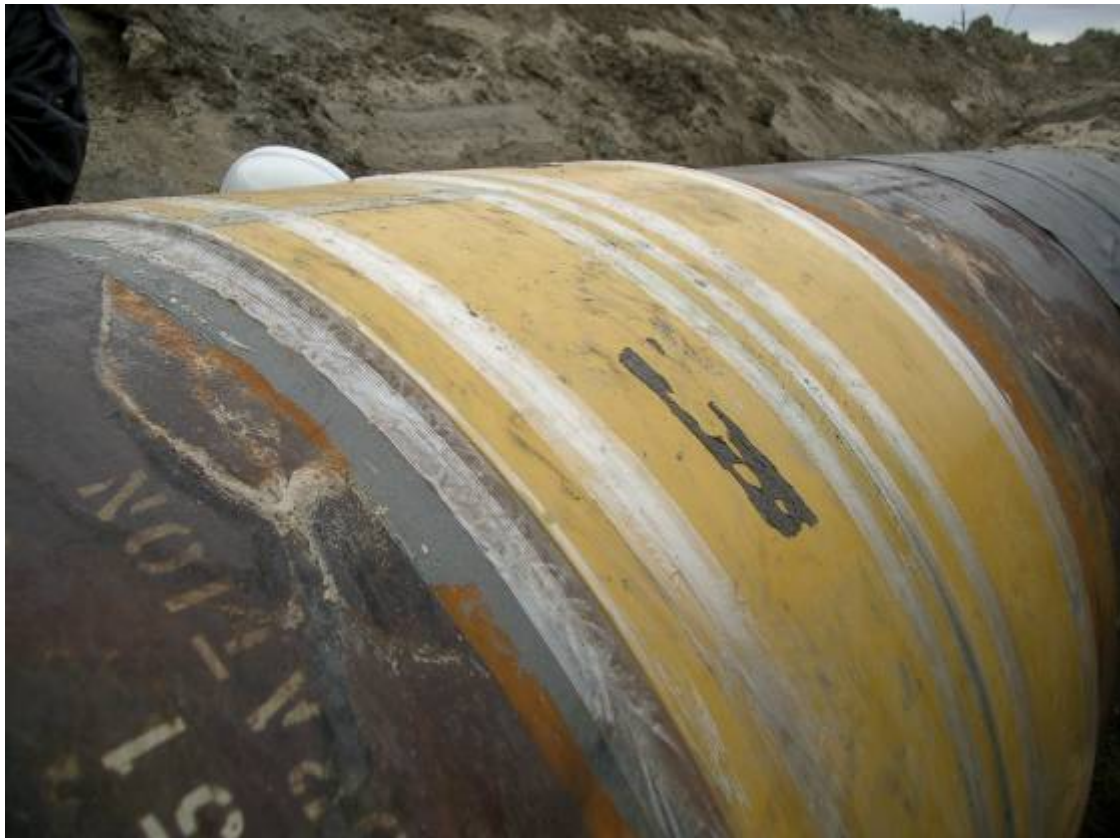
Figure 9 Example Repair Selection: Corrosion
