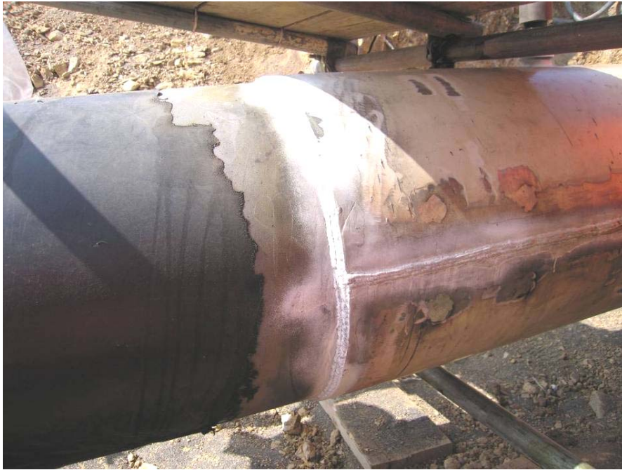
Figure 4 Close Fitting (Type B) Welded Sleeve
