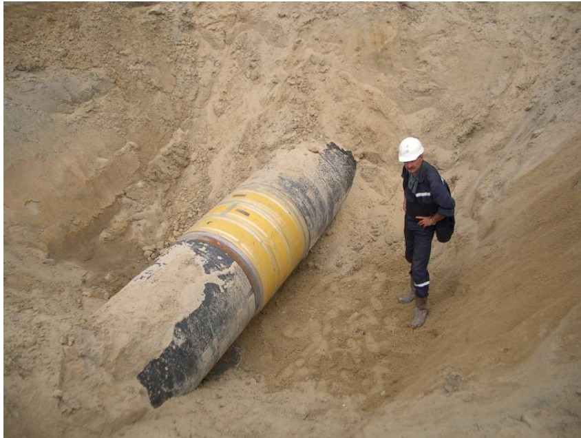
Figure 6 Composite Wrap Repair
