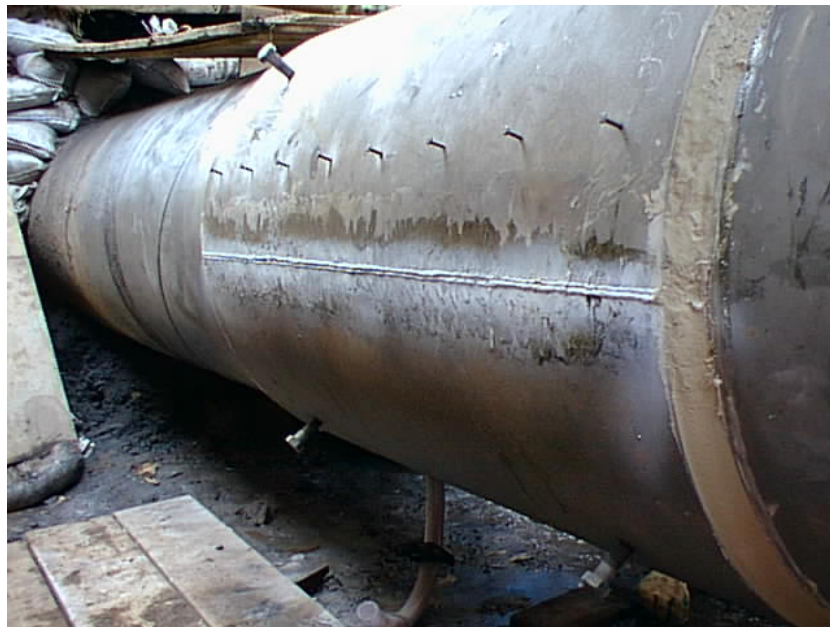
Figure 5 Epoxy Grout Filled Sleeve
