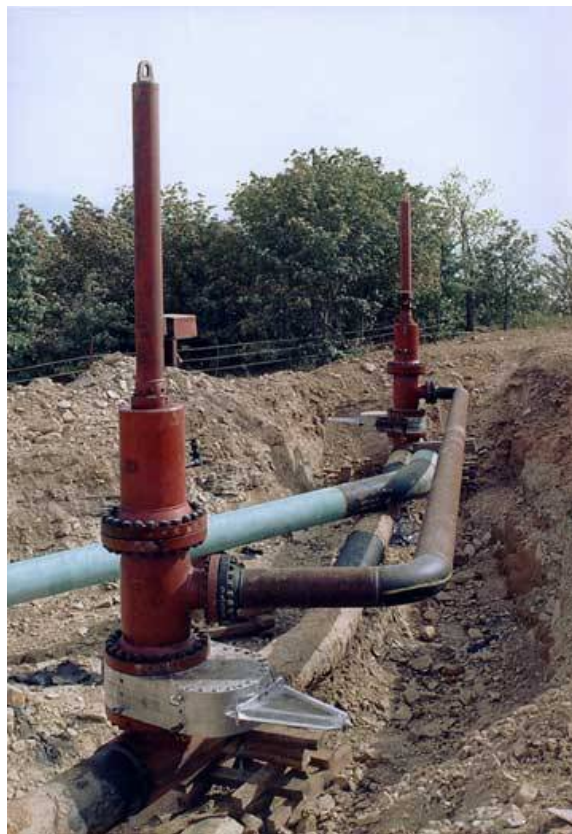
Figure 9 Stopple and Bypass (www.tdwilliamson.com)
