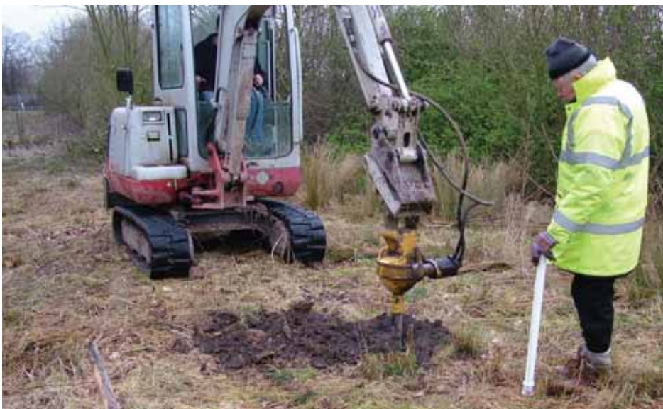
Burying the 'leak-tube' along the pipeline route.
