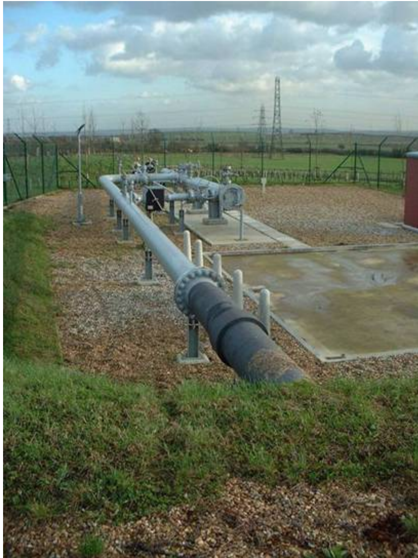
Figure 6 Pig trap and working area
