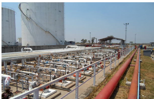
Figure 2. Harare tanks and pumps.
