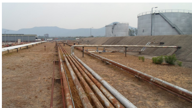
Figure 1. Feruka tanks and piping.
